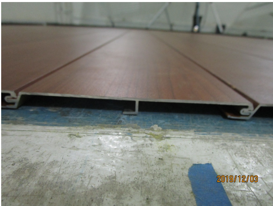
Figure 2 – Detail of tongue and groove joints
