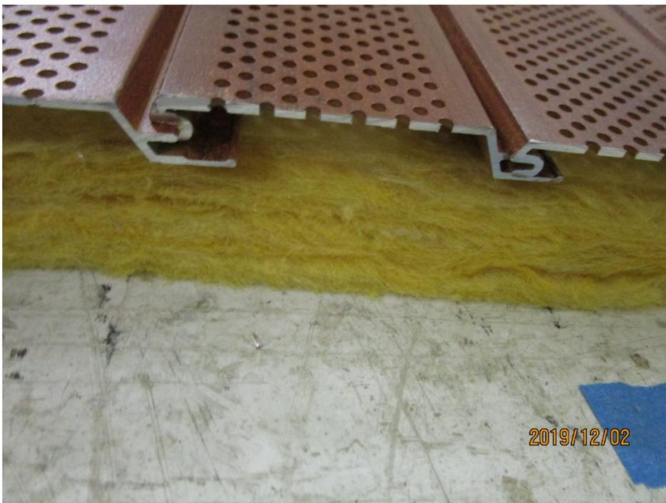
Figure 2 – Detail of tongue and groove design, plank joints
